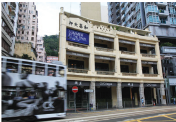
Figure 2 URA Johnston Road Preservation Project
