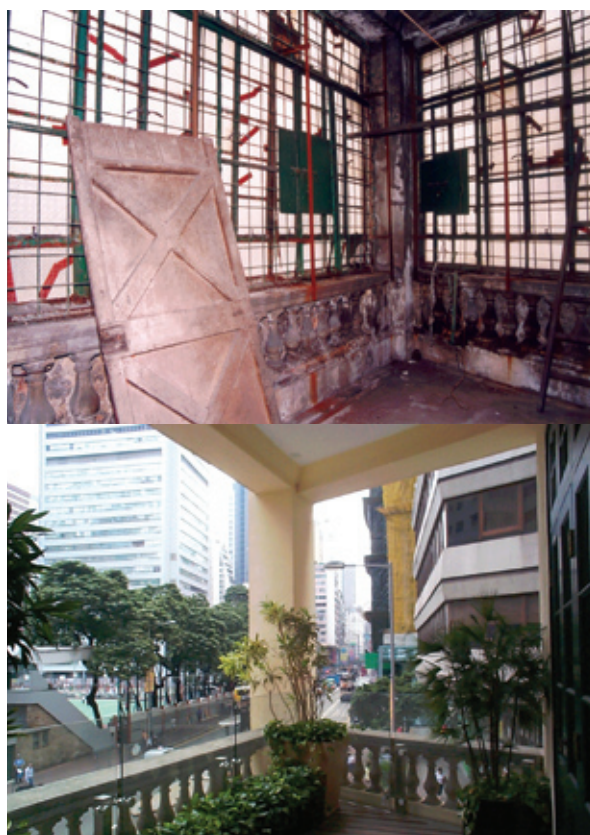
Figure 3 Opening up verandahs
