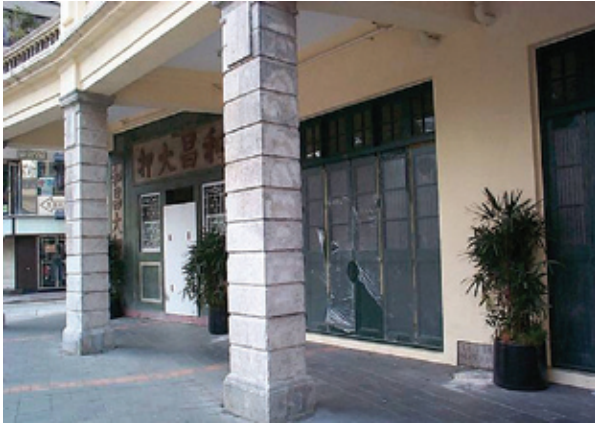
Figure 4 Restore granite columns
